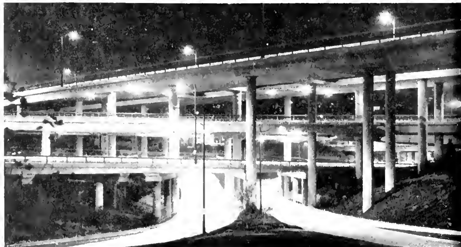
View of four level grade separation structure taken at night. On the lower level the light streaks on the right are approaching headlights and the fainter light streaks on the left are receding tail lights.
